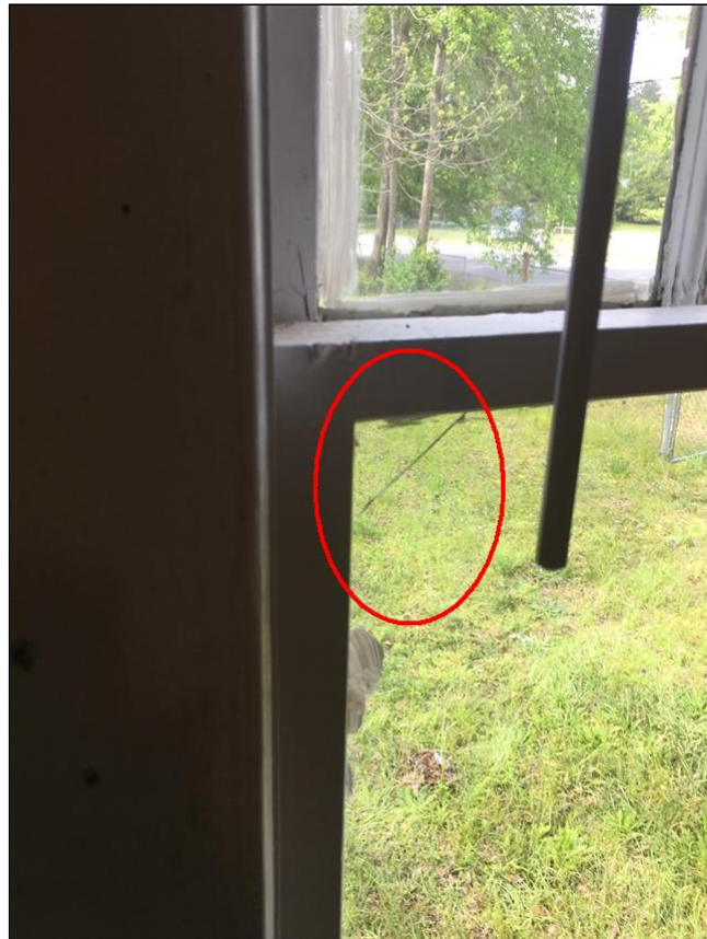
2.2 Item 4(Picture) Cracked window glaze
