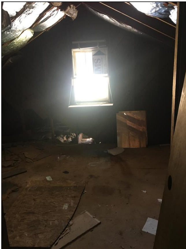
2.2 Item 7(Picture) Damaged window in attic
