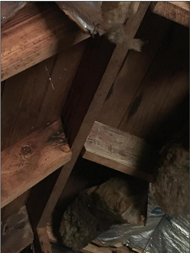
Rafters roof system
