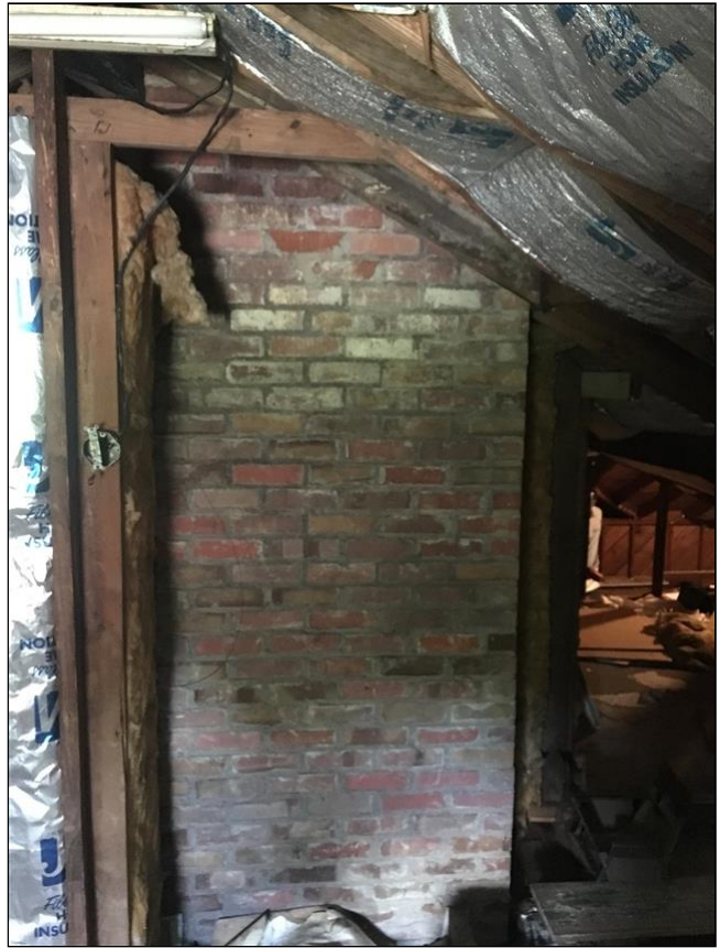
1.2 Item 4(Picture) Chimney chase in attic
