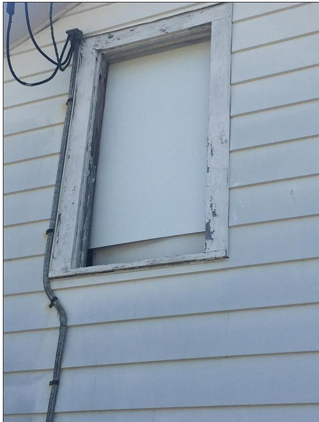
2.2 Item 8(Picture) Window missing
