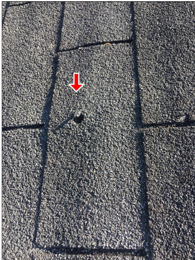
1.0 Item 6(Picture) Nail pops - can result in leaks
