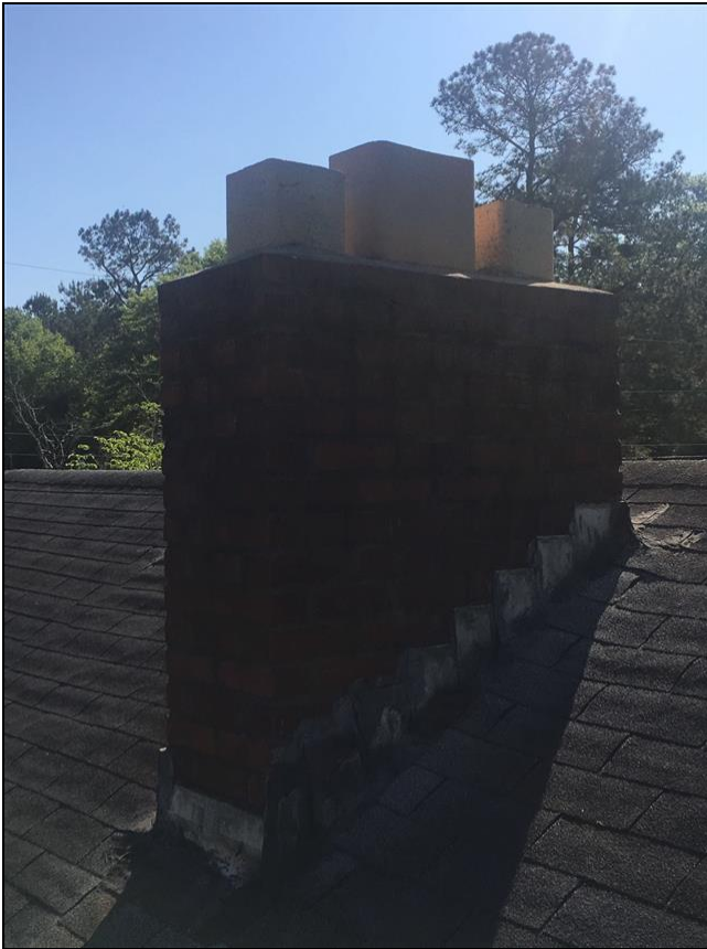
1.2 Item 1(Picture) Exterior chimney chase
