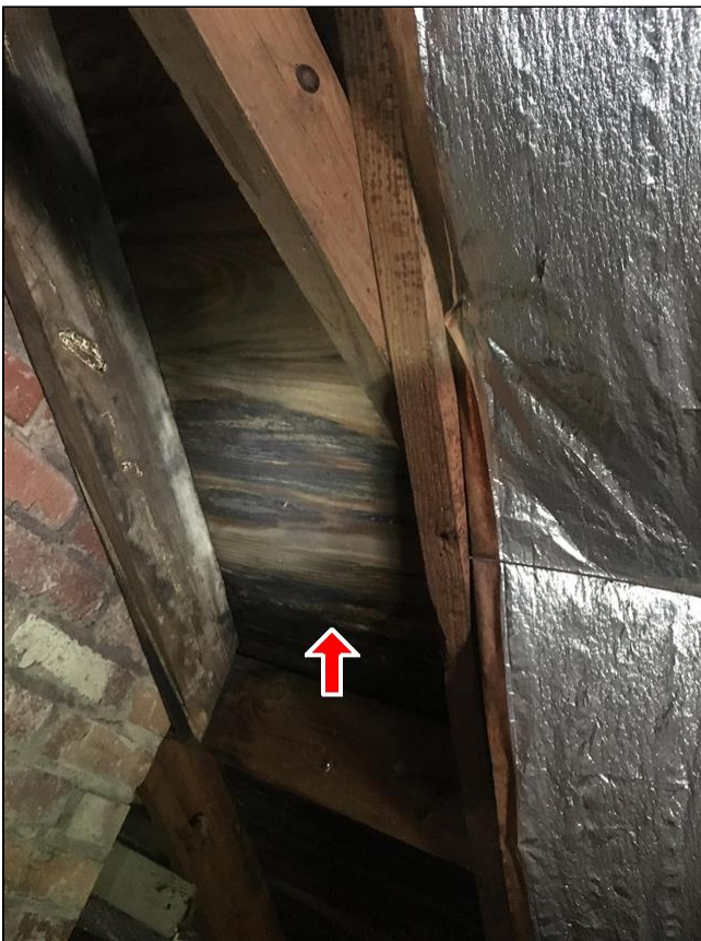
1.2 Item 5(Picture) Moisture stain near chimney chase in attic
