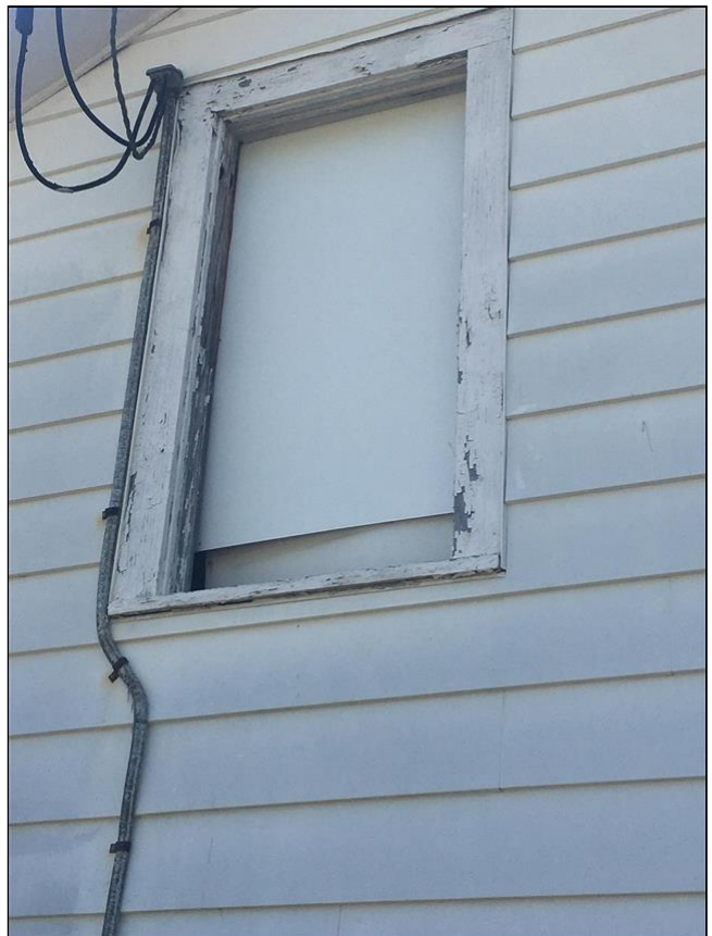
2.2 Item 8(Picture) Window missing
