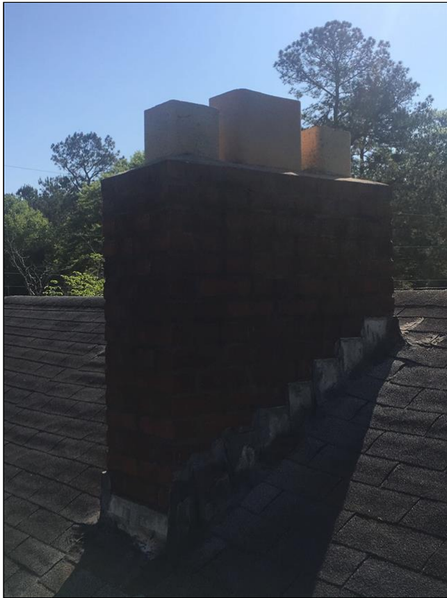
1.2 Item 1(Picture) Exterior chimney chase
