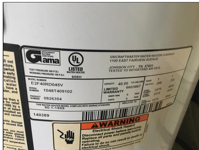
Water heater data label
