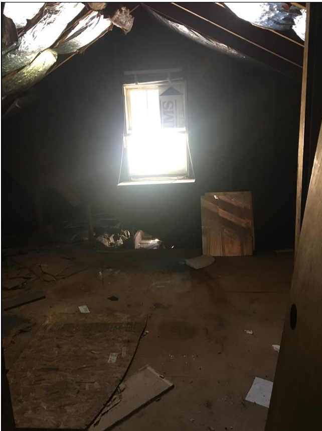
2.2 Item 7(Picture) Damaged window in attic
