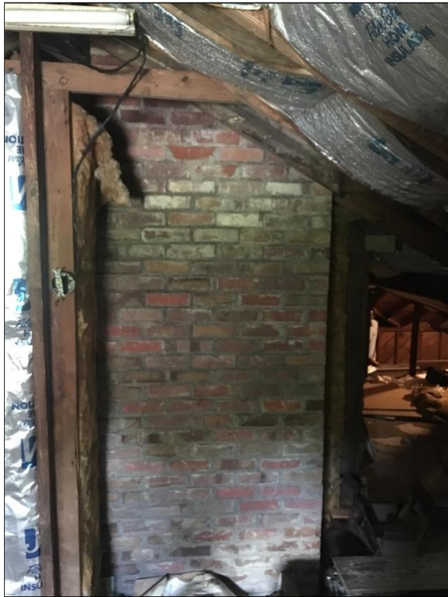
1.2 Item 4(Picture) Chimney chase in attic
