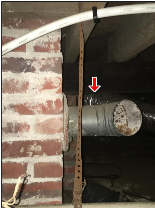
Apparent chimney clean out in crawlspace- see illustration
