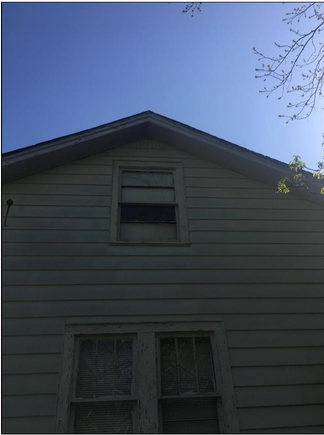
2.2 Item 5(Picture) Exterior view of missing window
