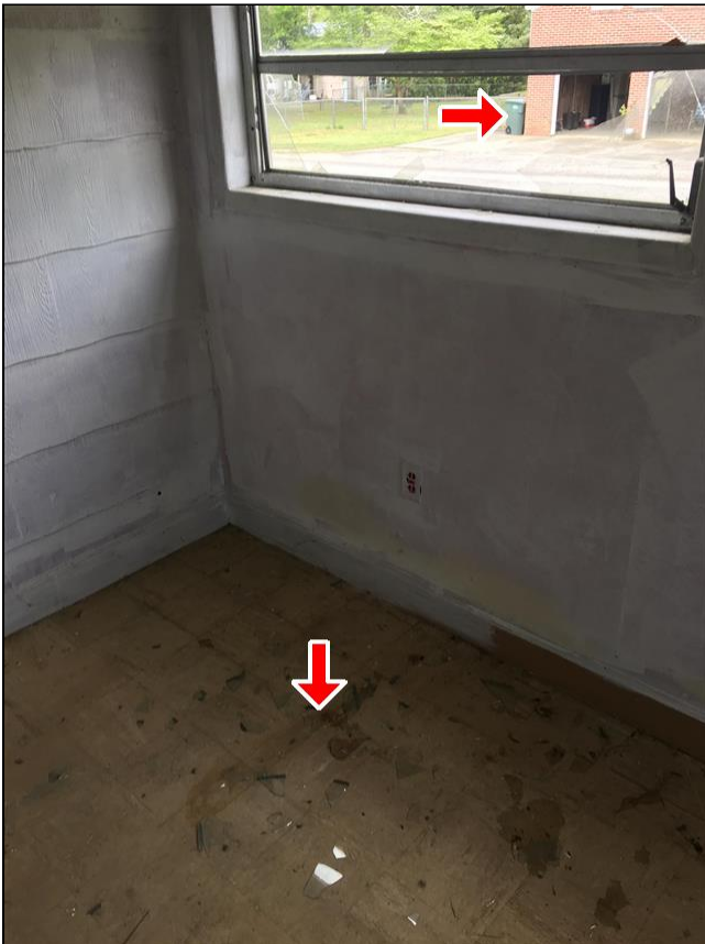
2.2 Item 3(Picture) Glass broken/shattered - on floor
