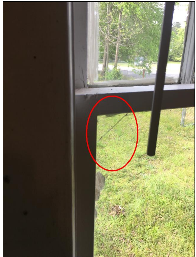
2.2 Item 4(Picture) Cracked window glaze
