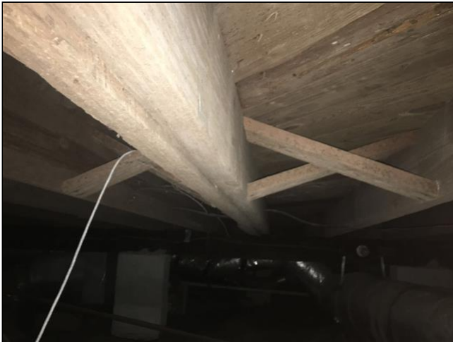
Joists in crawlspace
