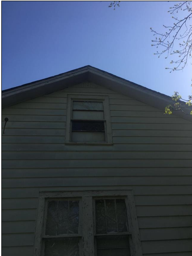
2.2 Item 5(Picture) Exterior view of missing window
