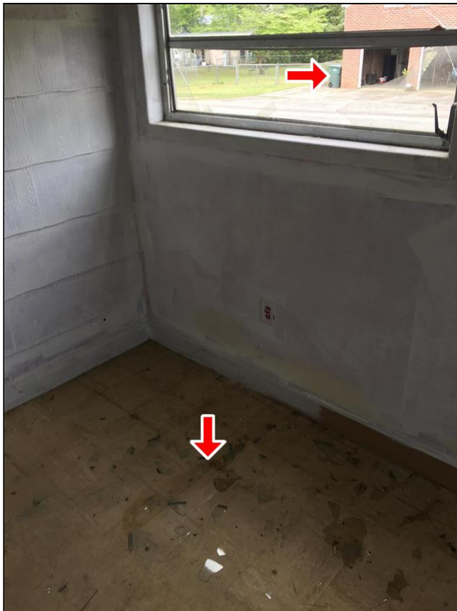
2.2 Item 3(Picture) Glass broken/shattered - on floor (2) Multiple windows missing; recommend installing
