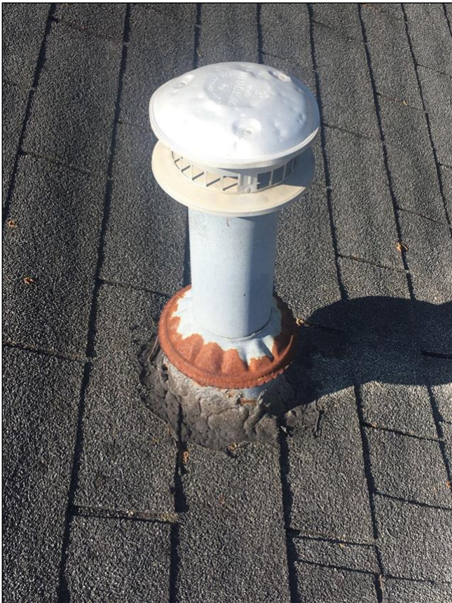
Metal flue - roofside
