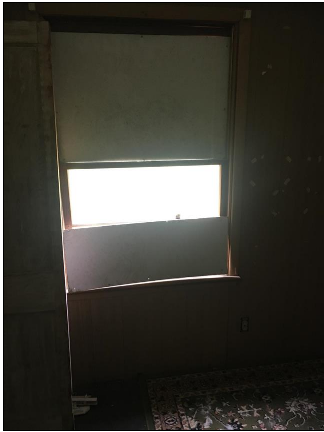
2.2 Item 6(Picture) Window missing
