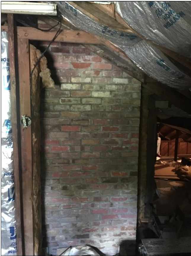
1.2 Item 4(Picture) Chimney chase in attic
