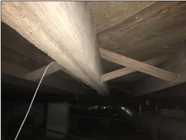
Joists in crawlspace
