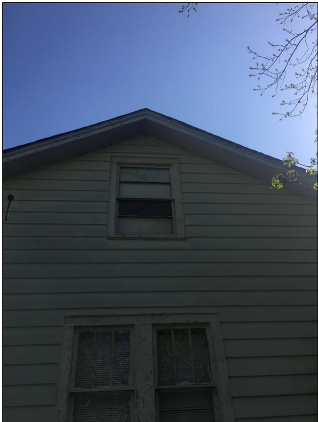
2.2 Item 5(Picture) Exterior view of missing window
