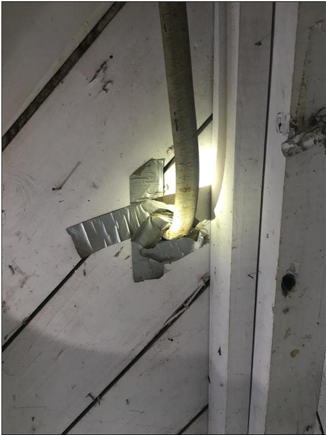
9.0 Item 2(Picture) Interior electric service wire not properly bonded; recommend repair
